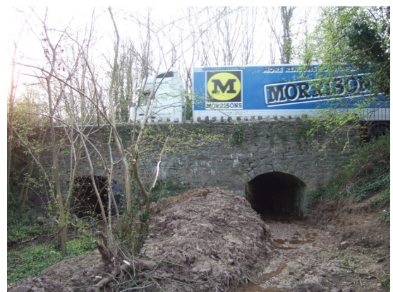
Newly cleared tramway tunnels under the A483
