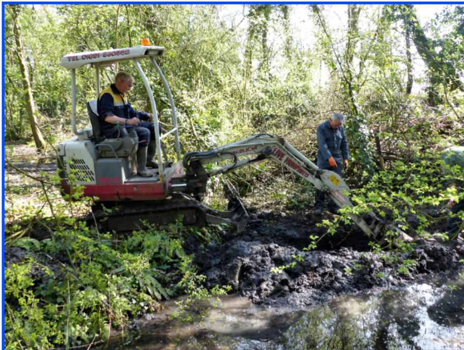
Revealing the drain under the embankment to the lower meadow
