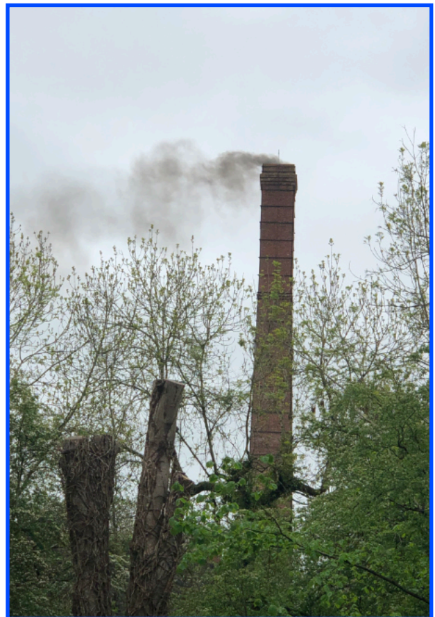
Smoke from the Hoffmann Chimney
