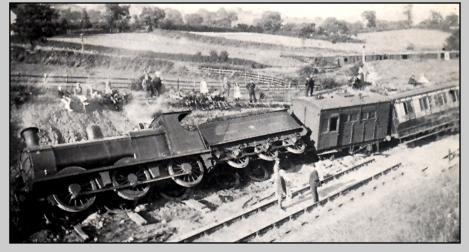
THERE was an accident at Wern Junction (near Carreghofa School) on 7 August 1908. A livestock train of Great Central stock was derailed as it left the Nantmawr line to join the new spur to Llanfyllin, just past the bridge under the canal. The engine fell on its side, and the track was badly damaged. At the inquiry excessive speed was blamed.
