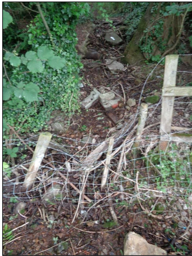
Figure 20: The majority of the site had well maintained fences and boundaries, but in some cases as here, repair work needs to be undertaken, this is near to where the stream enters the site. The rubbly nature of the embankment is apparent, presumably made of waste material from quarrying and household material.
